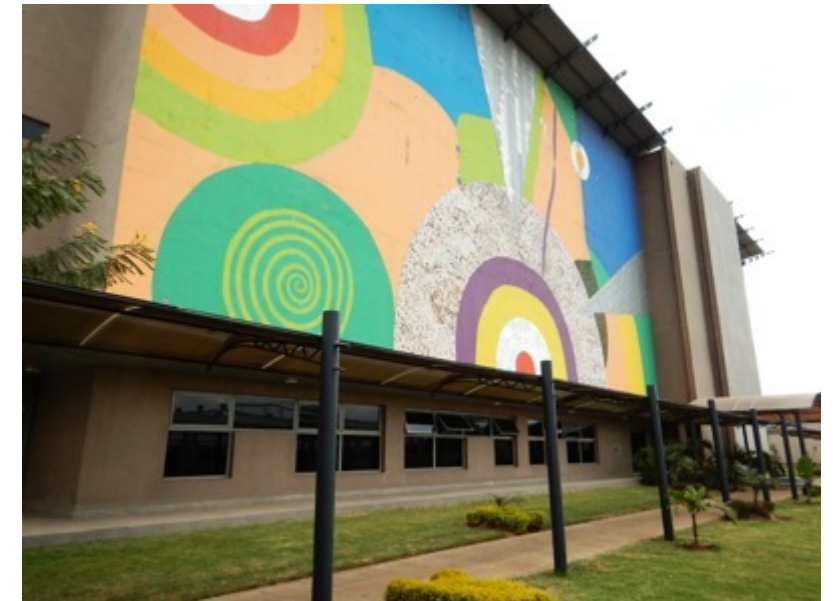
Data Centre, Nairobi, 2015
